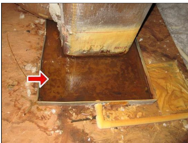
8.5 Item 3(Picture) Rusted drain pan
