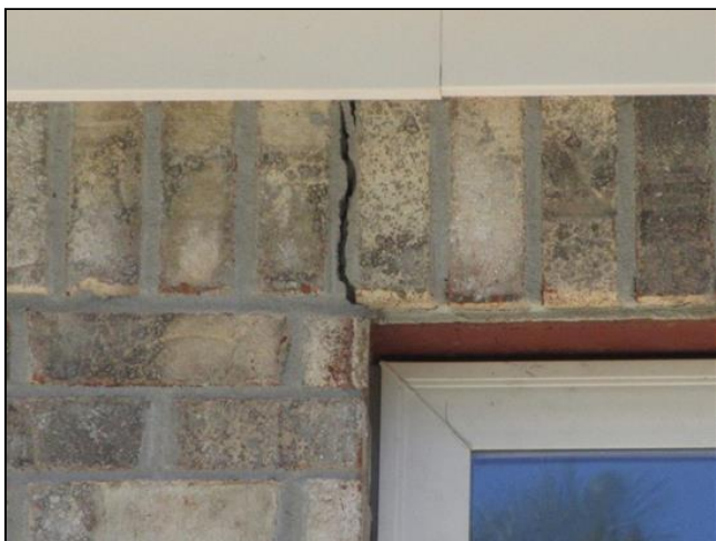
2.0 Item 3(Picture) Missing mortar
