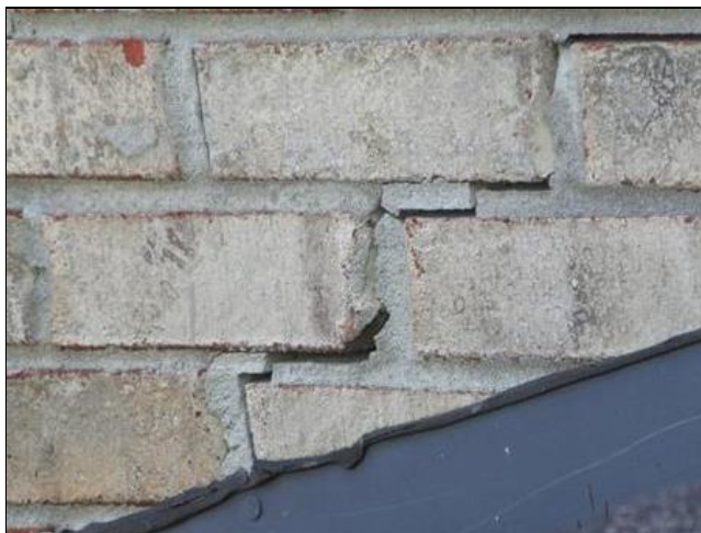
2.0 Item 2(Picture) Missing mortar
