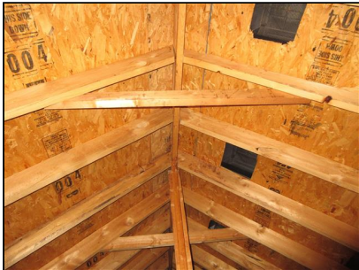
Pictures of Roof Structure/ Sheathing
