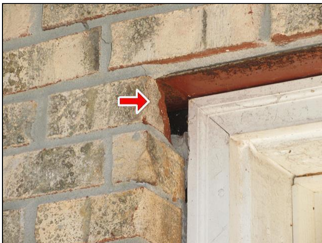
2.0 Item 1(Picture) Damaged brick
